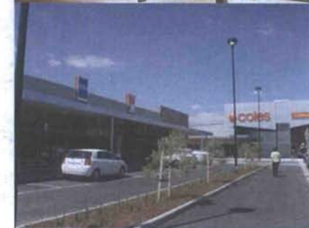
Figures 6 & 7: Well-articulated long facades with a range of materials and scale.
